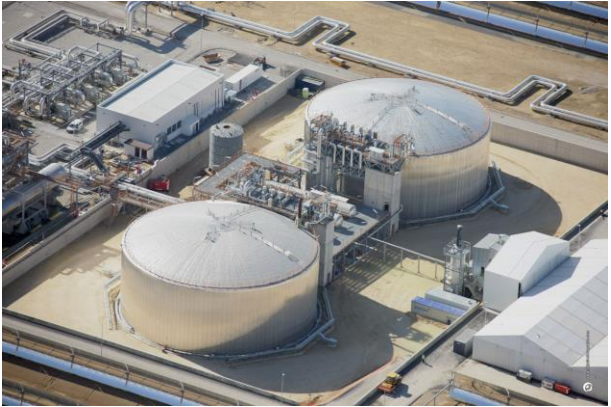
Molten Salt Tanks
