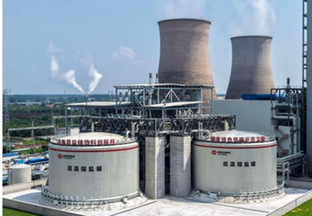
1GWh th molten salt in CHN Energy's 630MW coal power plant, China (2025)
